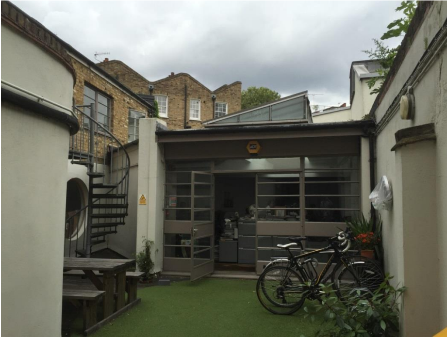
Image 3: View of existing part single/part two-storey building
